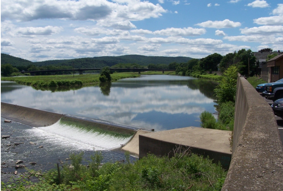
(The Chase-Hibbard Dam in Elmira keeps river levels high enough to provide drinking water for more than 65,000 Elmira Water Board customers)
